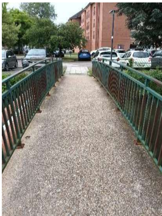
Figure 19 : Garde-corps corrodés
